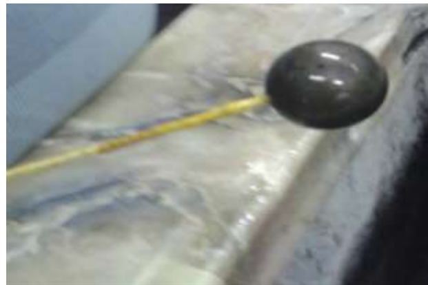
Figure 4. Roughened surface by corrosion
